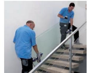
**i** Suction pad ø 120 mm · Number of suction pads 3 · suitable for Glass · suitable for Plastic · suitable for Metal · suitable for Coated Wood · suitable for Marble / Stoneware · with CE sign
